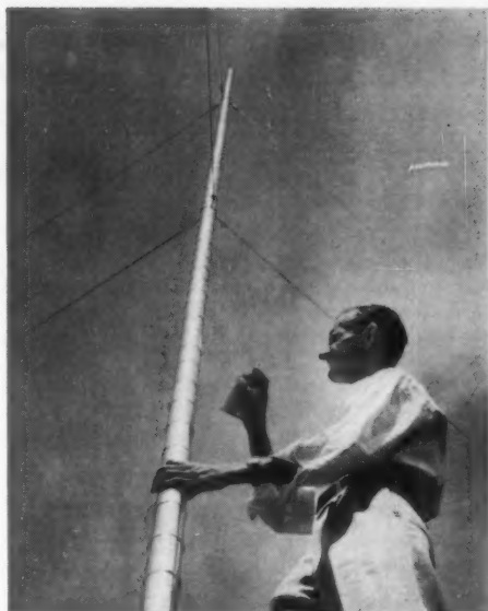
Here W2JTJ is touching up a spot on his antenna he missed with the aluminum paint the first time around. A lot of thought and libation went into the construction of this vertical.
